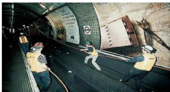
Figura 10 – Posa in tunnel metropolitana -
